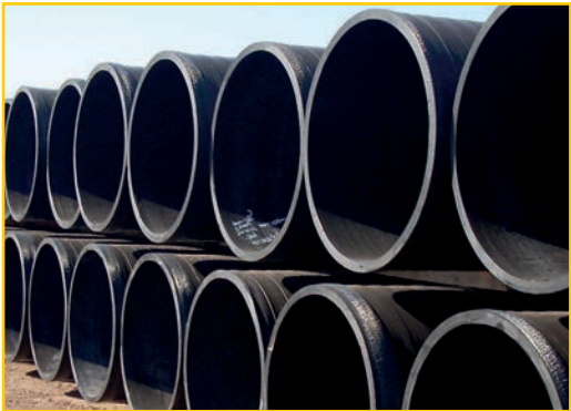
Storage on site
