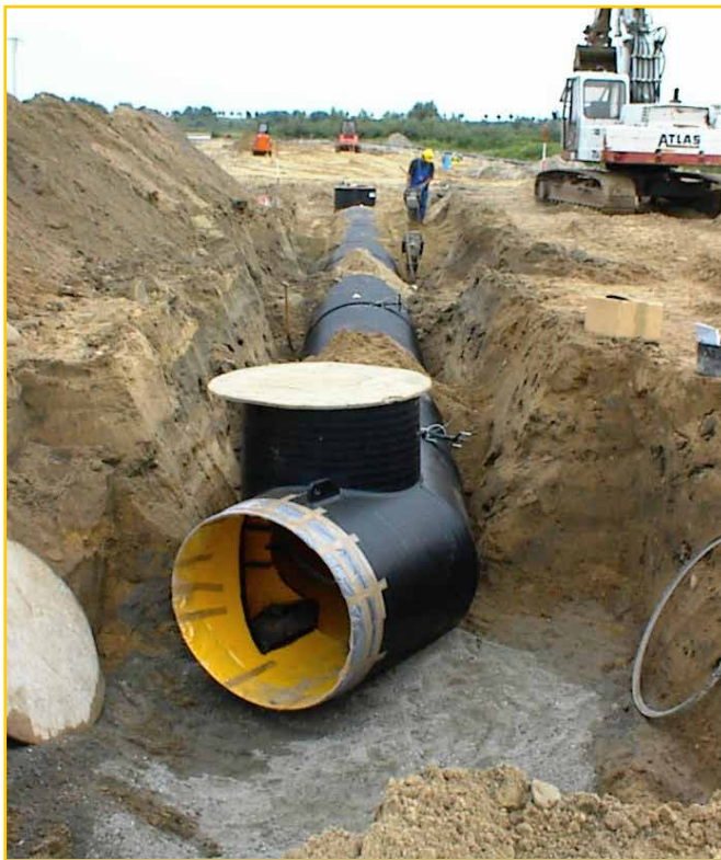
Installation of tangential manhole based on compacted soil (crushed stones)
