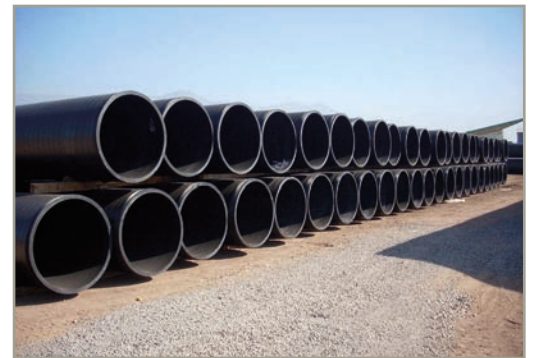
Storage on site
