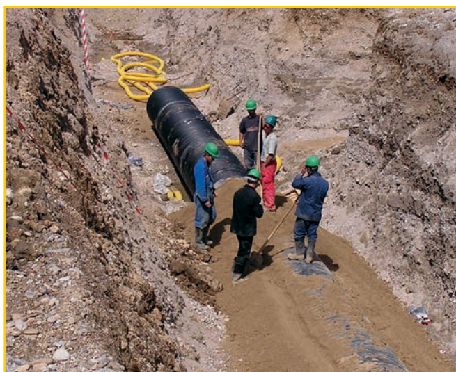
Compaction of main backfilling
