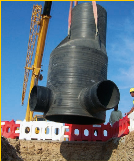
Manhole transportation on site
