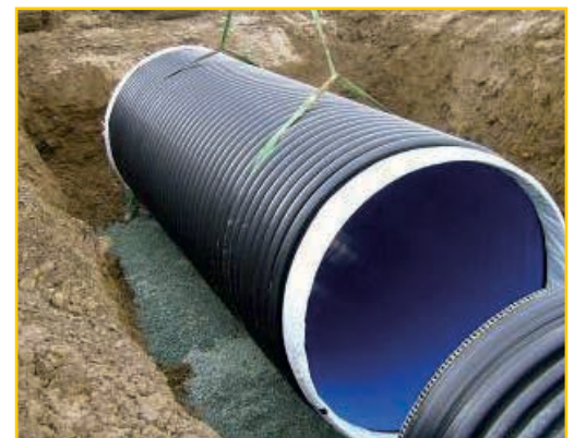
Placement on bedding material
