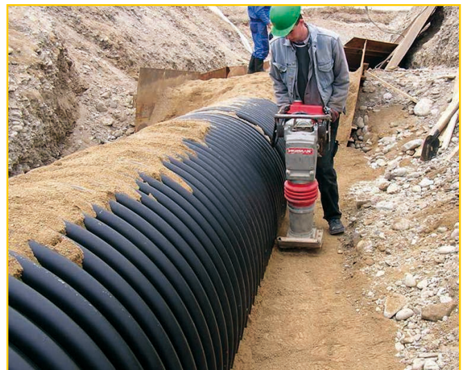
Compaction work with a vibratory plate
