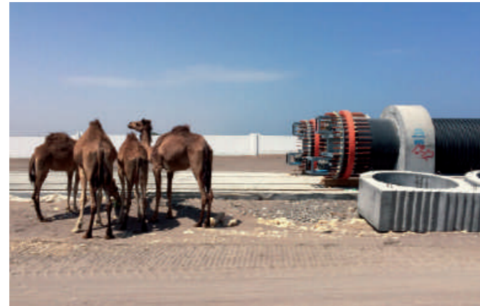
Pipe of DN/ID 2000mm (79") installation in a hot environment
