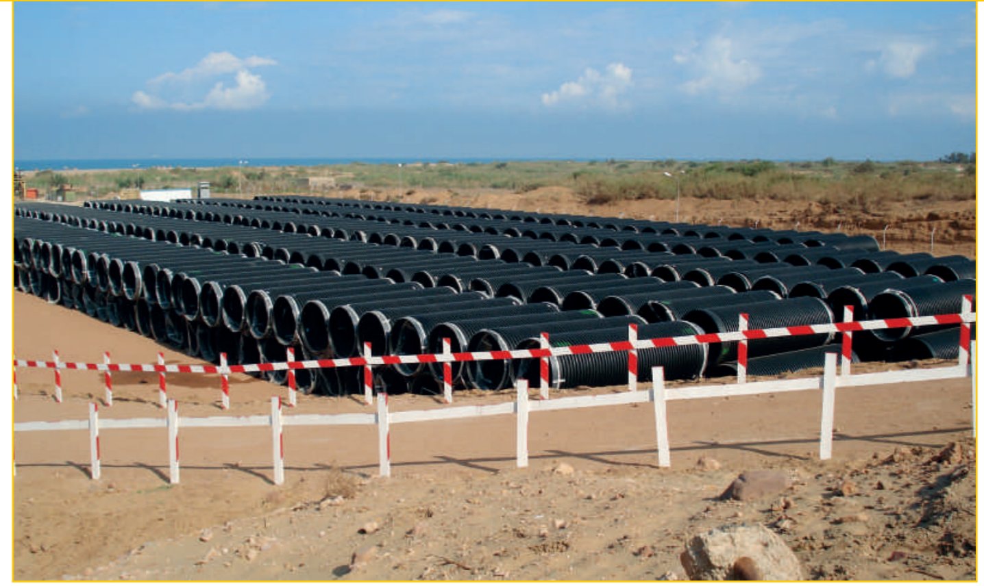
Open storage of pipes DN/ID 1600mm (63")
