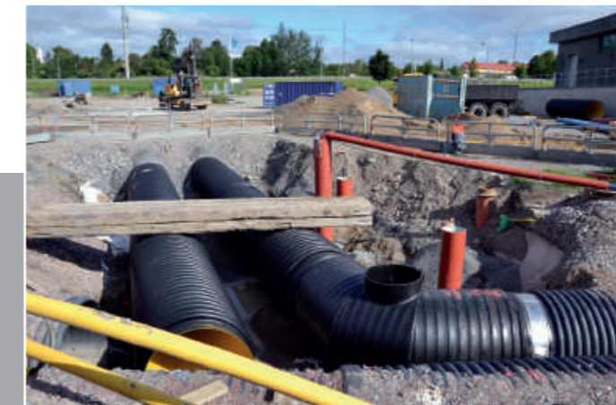
Fire fighting water tank
