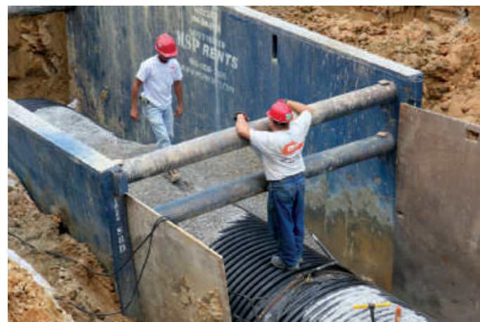
DN/ID 2200mm (87") pipe installation
