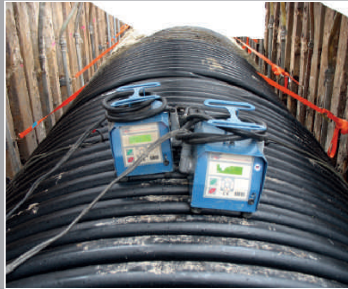
Electro-Fusion joint DN/ID 1800mm (71")
