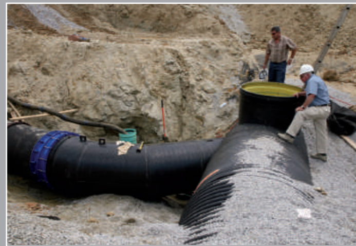
Installation of pipes DN/ID 2000mm (79"), with manhole & bench
