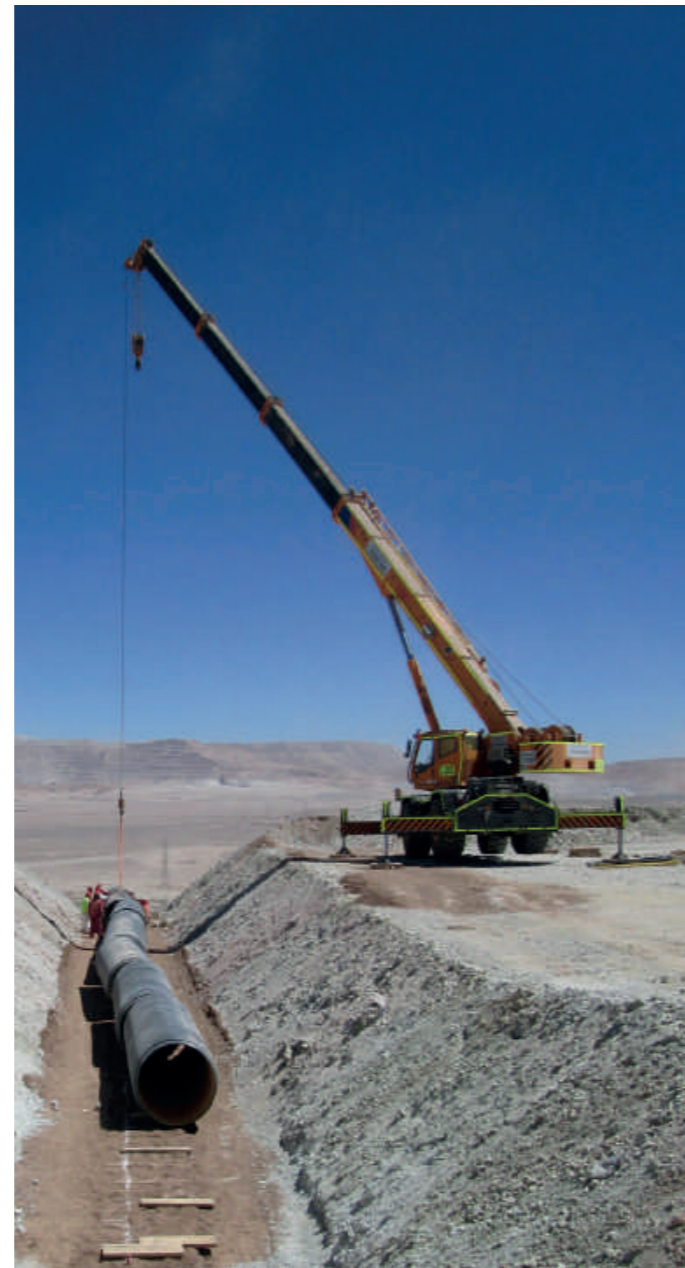
Installation of pipes DN/ID 1800mm (71") in a mining project for slurry
