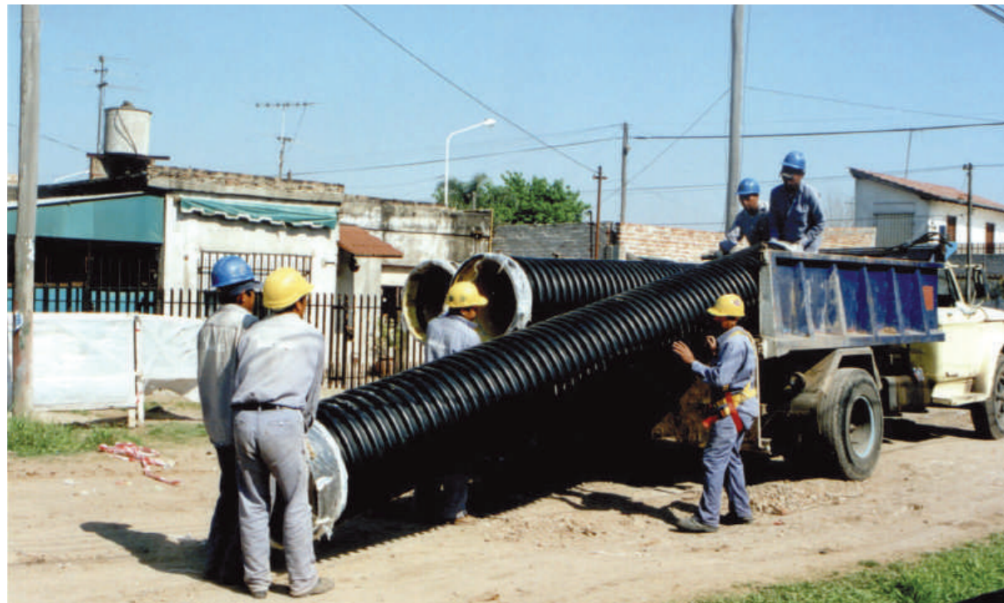
Light weight pipe - Manual unloading of a pipe DN/ID 600mm (24")
