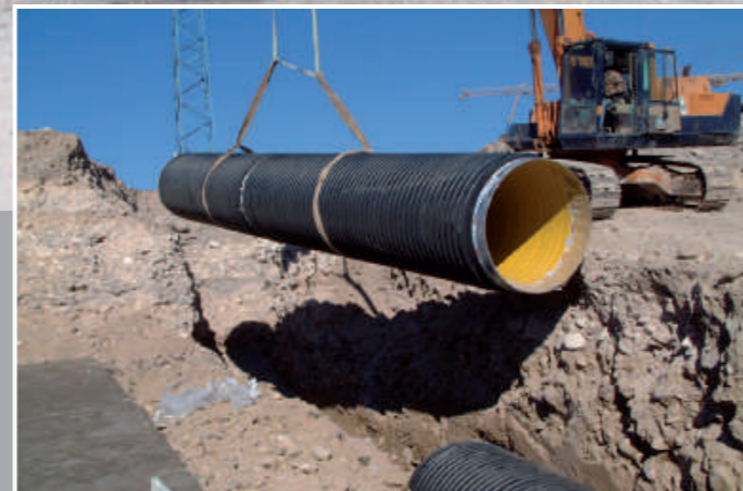
Installation of two pre-jointed pipes DN/ID 1600mm (63")
