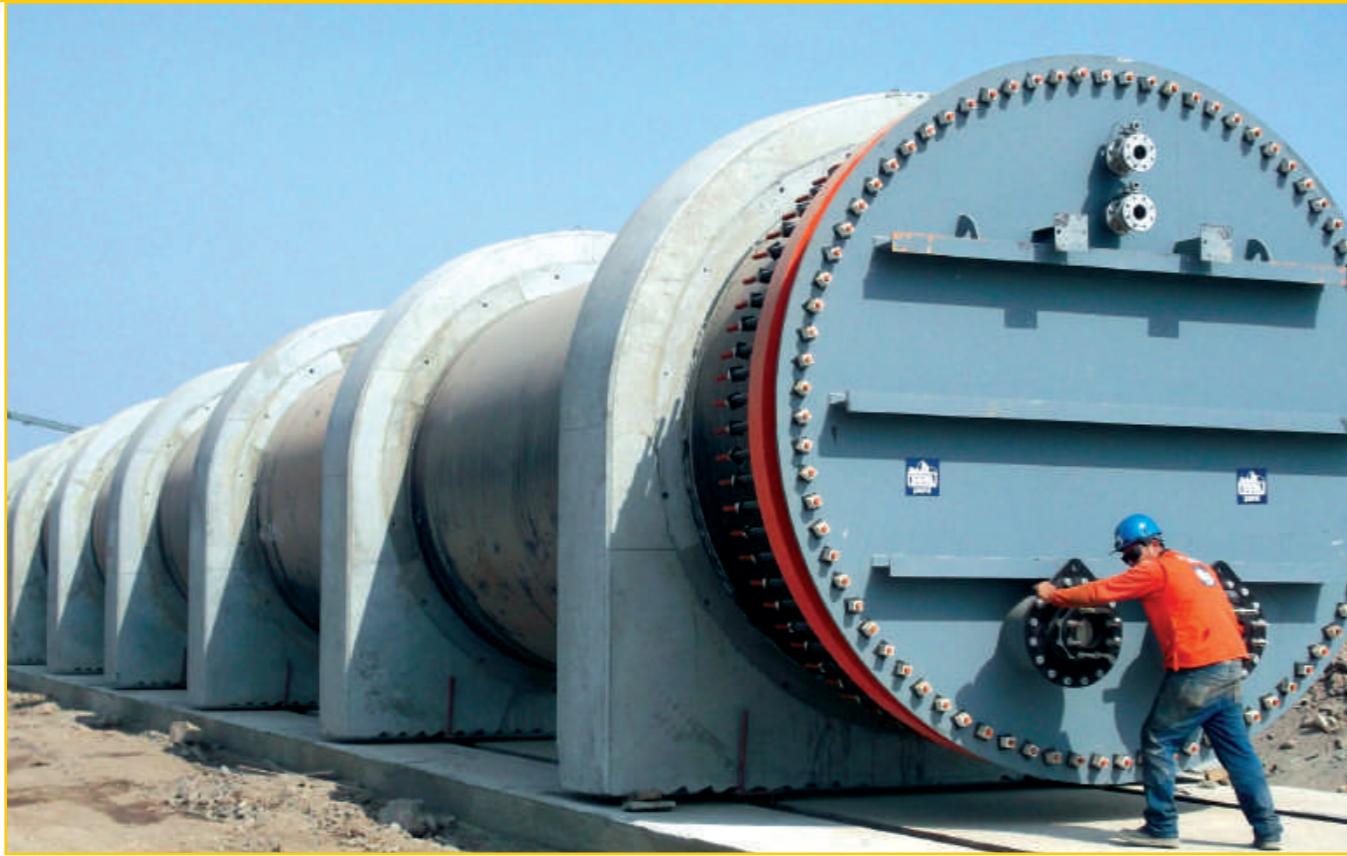
Preparing an outfall pipeline string DN/ID 3000mm (118")
