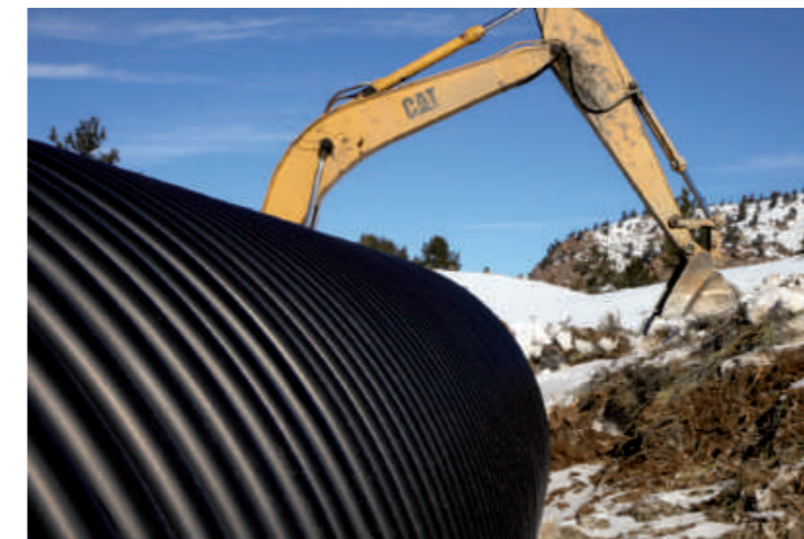
Installation of pipe with DN/ID 1600mm (63") during low temperature
