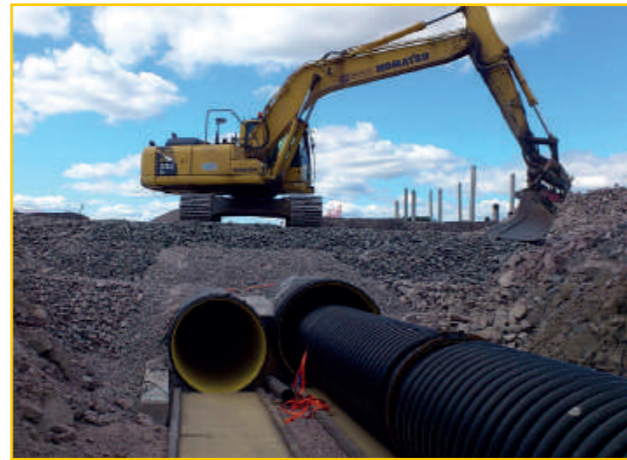
Installation of two pipe strings DN/ID 1200mm (47") and DN/ID 1400mm (55")
