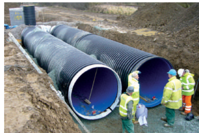
Installation of stormwater system DN/ID 1800mm (71")
